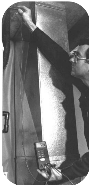
FIGURE 50 TEMPERATURE RISE MEASUREMENT
