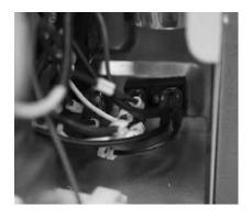
7. Locate high voltage wires and connect the high voltage ballast wires to the line voltage wires from the plug, using the supplied splice connectors.
