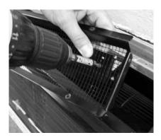
3. Secure PTAC unit to the bottom side of fan guard screen. When reattaching fan guard screen check for fan blade clearance.
