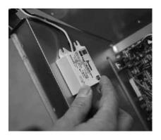
5. You can secure the ballast with either double stick tape or with supplied screws.
