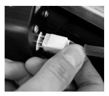
10. Connect lamp cord to lamp. If necessary drill 1/2" access hole to create a pass-through for lamp cord.
