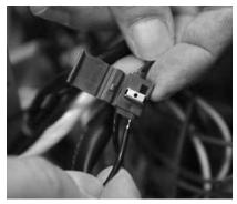
8. To use the wire tap splice terminal, first place around line voltage wires, then insert ballast wire, and press firmly. White to white and black to black. Tuck wiring from PTAC unit safely around the sheet metal and into the high voltage control panel.
