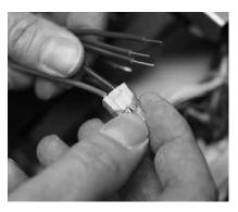
6. Using supplied wire nuts, attach wires from cell to wires from ballast. Matching blue to blue and red to red.
