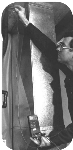
FIGURE 48 TEMPERATURE RISE MEASUREMENT
